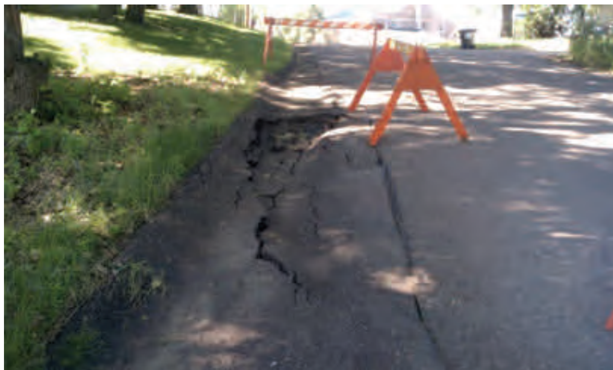
Road damage due to heavy rainfall in June
