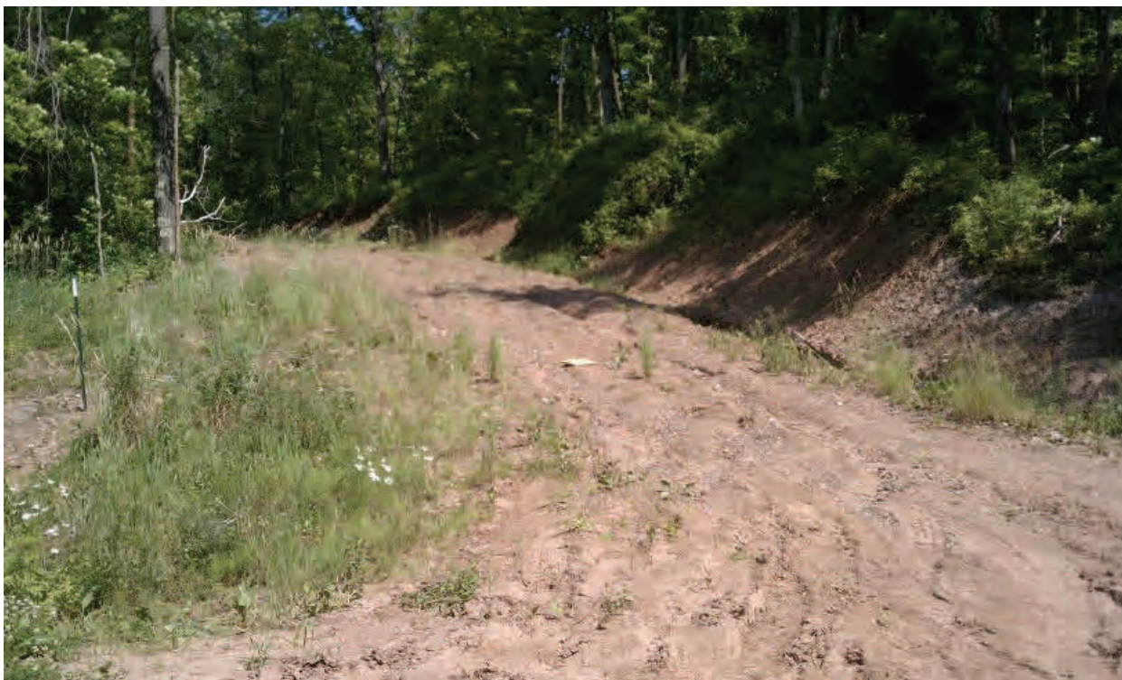
Washed out road/driveway
