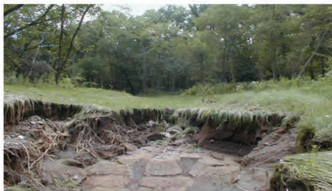
Figure 1. Much of the material eroded from this sediment-filled channel constructed during 1930s will enter Big Rock Creek on its way to the St. Croix River. (Photo by Keith Zygowicz, NRCS, Balsam Lake, WI)
