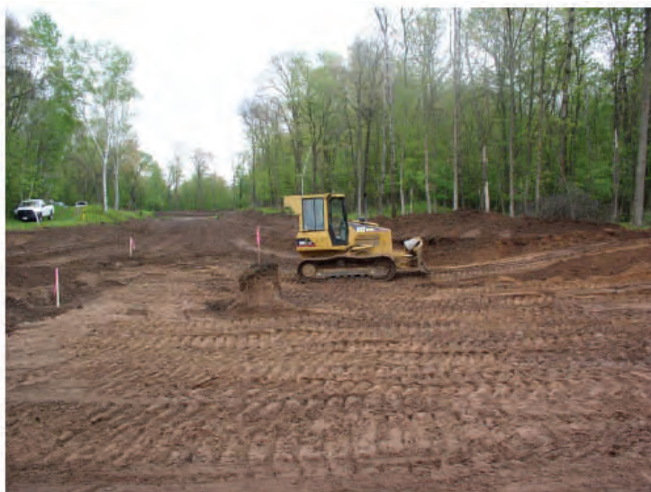
Figure 2. Sediment removal and channel re-grading. Approximately 3.5 feet of sediment was removed at this location. (Photo by Keith Zygowicz, NRCS, Balsam Lake, WI)
