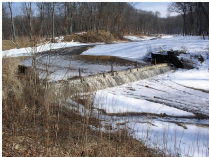
Figure 3. Runoff controlled at upper end of project site by reconstructed channel and structure. (Photo by Keith Zygowicz, NRCS, Balsam Lake, WI)
